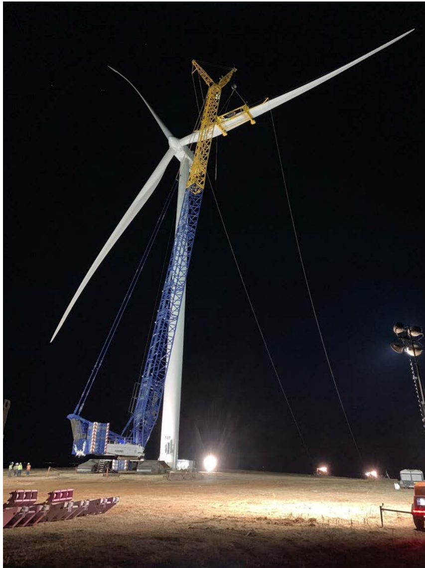
Last blade being installed – November 11, 2020
