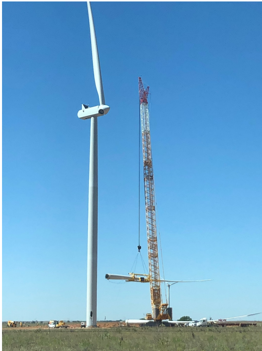
Blade install – June 8, 2020
